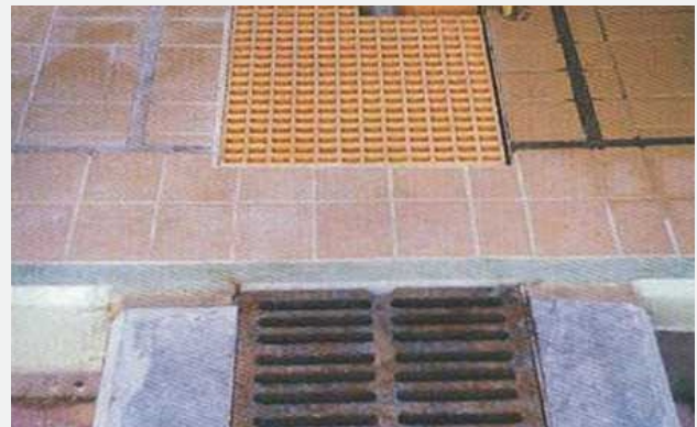
Corroded Steel Grating Vs GRP Moulded Grating
