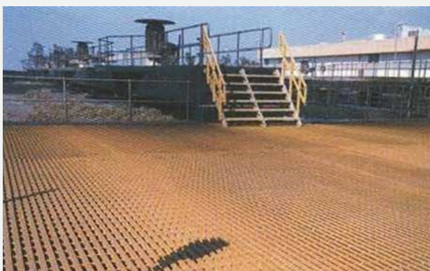
Pultruded Grating in sewerage Treatment Plant
